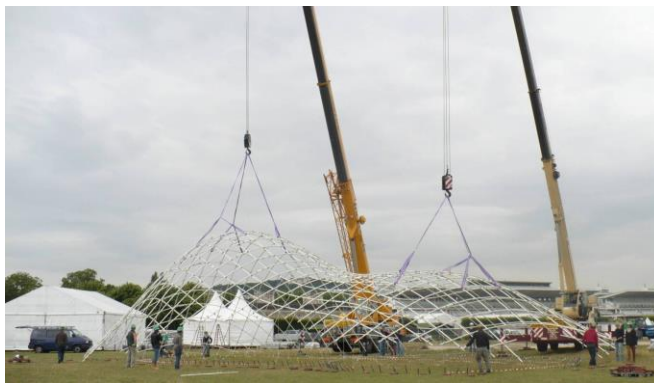
Fig 6. Positioning of the grid with crane
