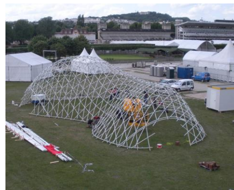
Fig 7. Gridshell anchored and braced
