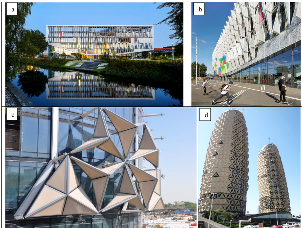
Fig. 1. Examples of Adaptive Solar Façade (ASF) as an energy-saving design concept for a sustainable future (a, b) SDU University of Southern Denmark Campus Kolding, Denmark, by Henning Larsen Architects, 2014 (c, d) Al Bahr Towers complex in Abu Dhabi, United Arab Emirates, by: Aedas Architects, 2012 [16].
