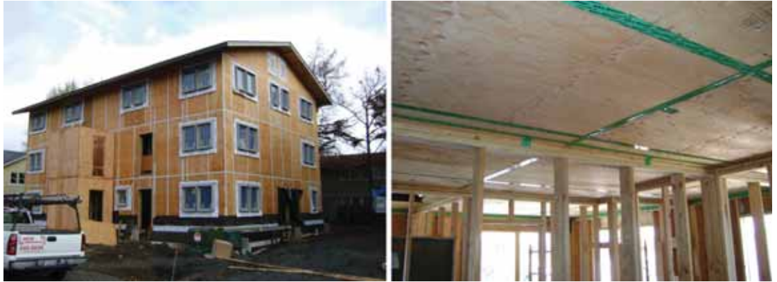
Figure 4: Taped plywood seams throughout PH.
