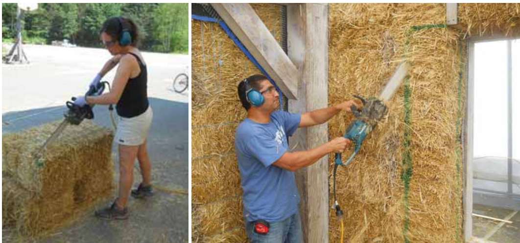
Figure 1: Squaring of bales (prior to installation) and beveling of window wall edges with chain saw.
