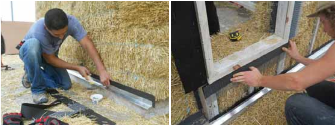
Figure 2: Application of air-fins, flashing, and metal lath at critical transitory locations along the wall plane.
