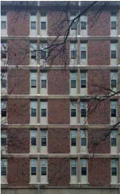
Figure 2: Thermal bridges with exposed concrete.
