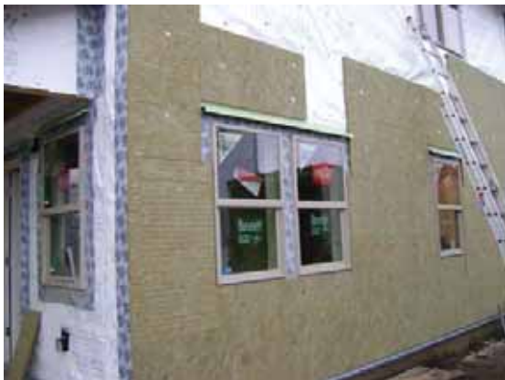
Figure 3: Continuous insulation over WRB on PHIF.
