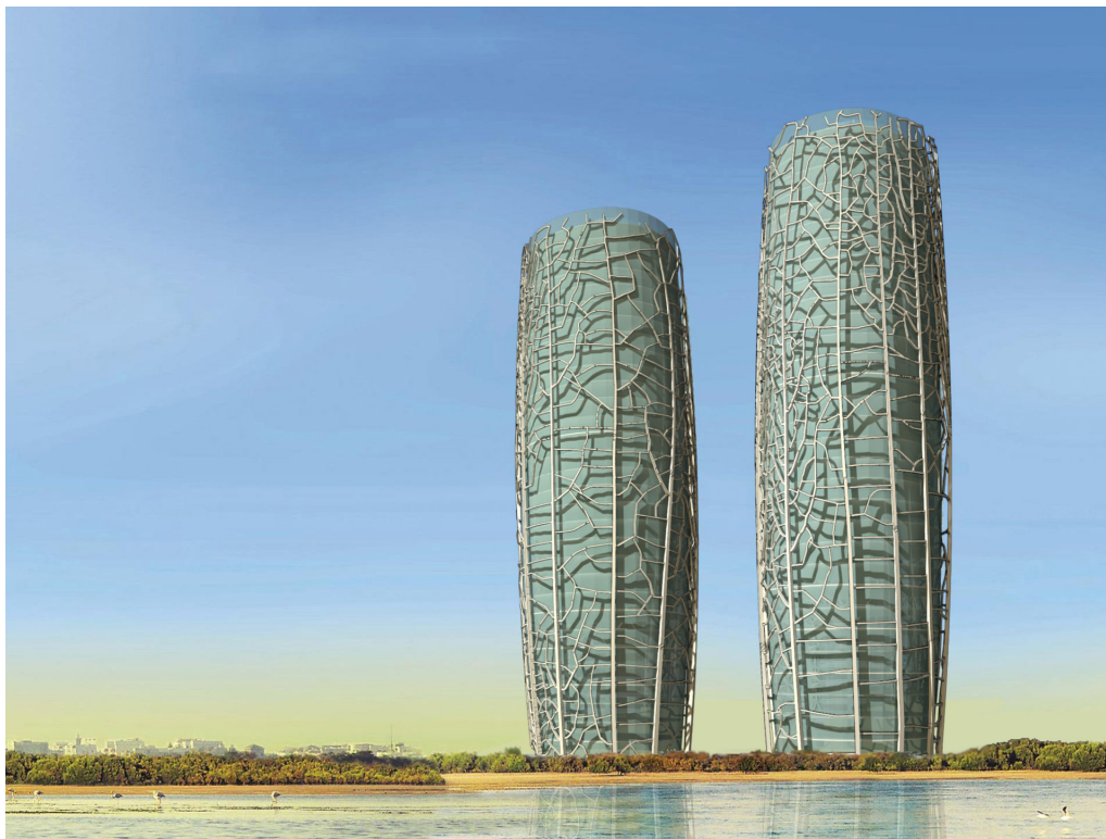
Figure 7 A rendering of the structural façade system generated by the leaf venation algorithm.
