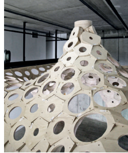
Fig. 4: The upper bound geometry skips continuity at the connection of the voussoirs due to the requirement for the milling operation to have a flat surface.
