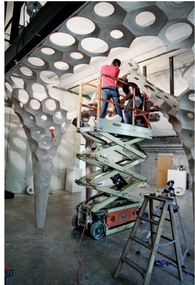
Fig. 11: Assembly of the vault.
