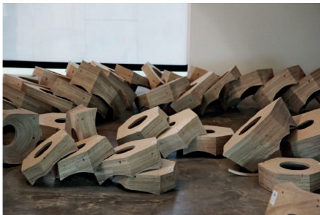
Fig. 10: Various unique voussoirs that compose the vault.
