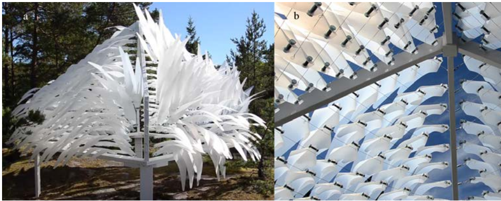
Fig. 5. (a) The passive movement caused mainly by the wind; (b) Close-up of the kinetic mechanism.
