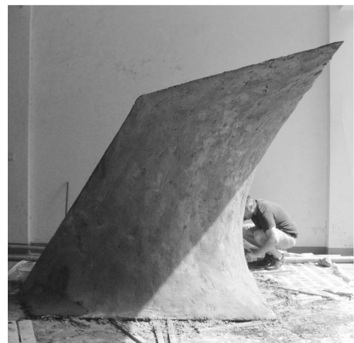
Fig. 18. A smooth poly-hypar surface made with ferrocement. Six hypar modules were welded from steel rebars, assembled into the skeleton of a cantilevering shell (above), wrapped by a steel mesh (middle), and then covered with concrete (bottom).
