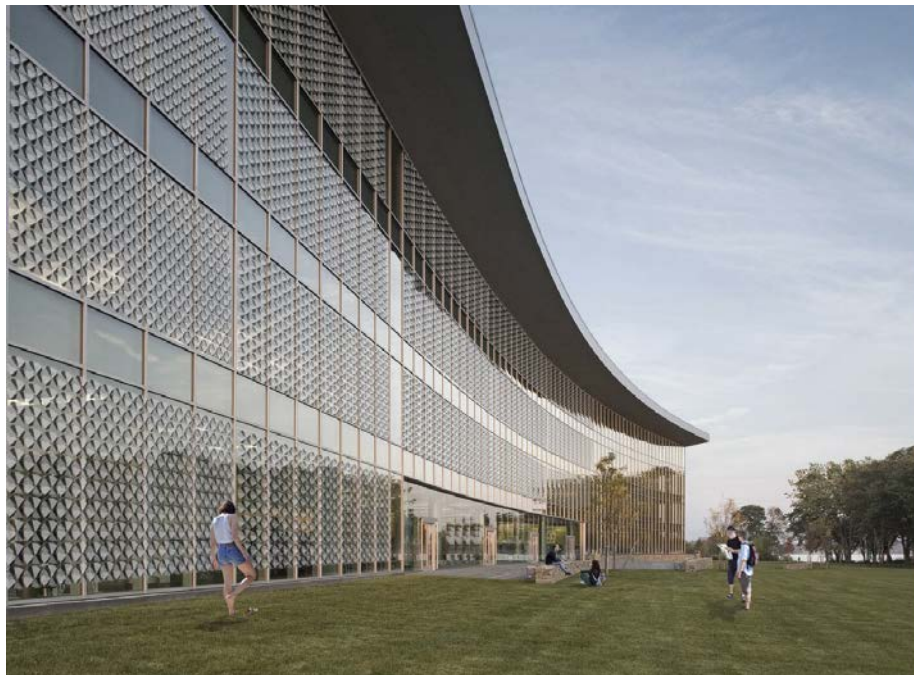
Fig. 10. Exterior rendering of proposed flexagon responsive shading system
