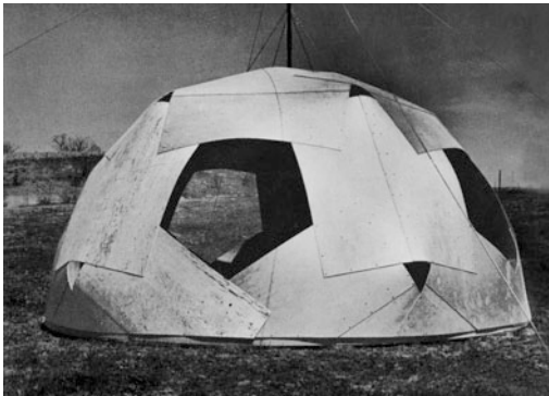
Fig. 1 Two-frequency geodesic plydome in Des Moines, Iowa, 1957. The hemisphere spans 7.3 m and is made out of marine plywood sheets with a thickness of 6.4 mm. (Marks 1973, p. 210)
