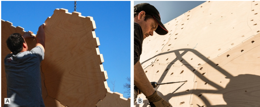
Figure 10. A: Assembly of a structural plywood plate. B: The plates are fixed and held in place through the crossing screws.
