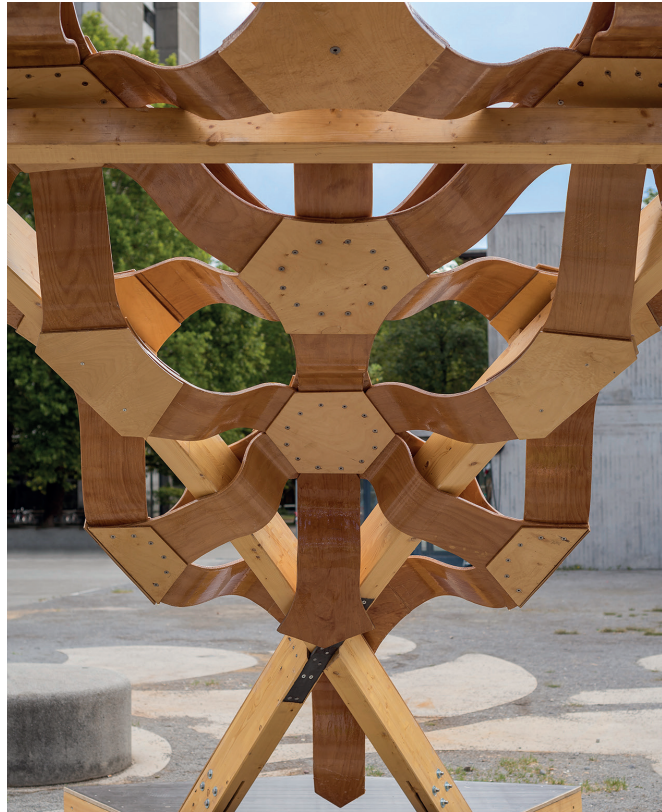
24 Detail of the shell connection with the beam
