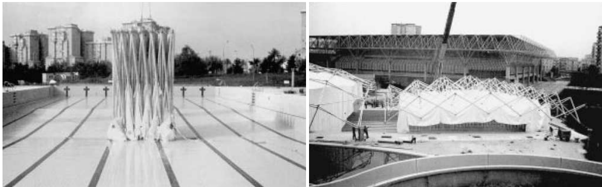
Figure 12 - F. Escrig , deployment of roof elements over a swimming pool in Seville.
