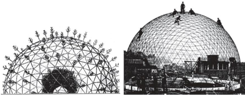
Figure 42: Dome-forming node-and-rod structures in nature and in architecture - Silicate skeleton of a radiolarian and first planetarium of Zeiss, Jena
