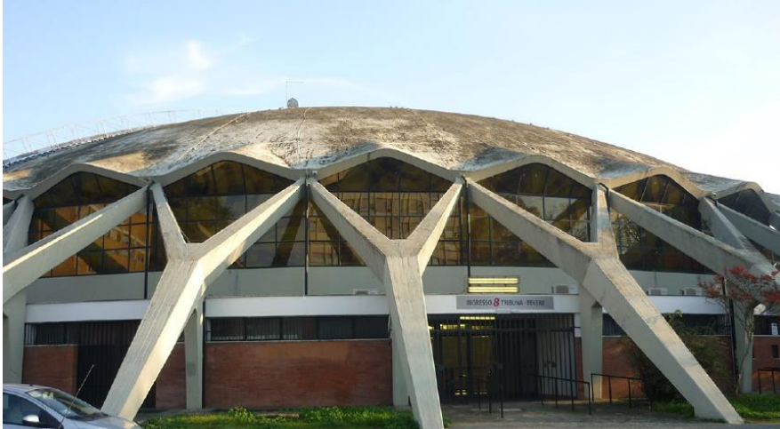
Figure 69: Y-shaped buttresses supporting the roof
