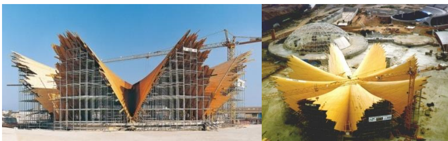
Figure 94: The formwork of the Submarine Restaurant of L'Oceanogràfic
