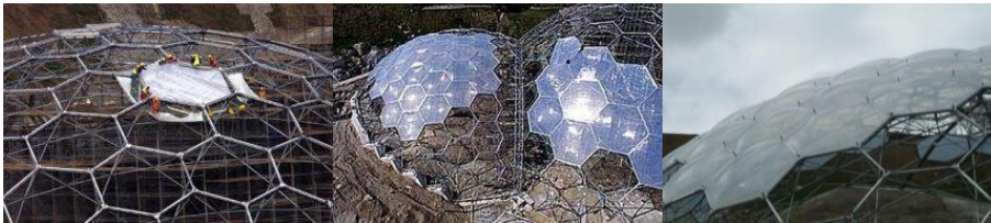
Figure 135: The hexagonal structure of the biomes
