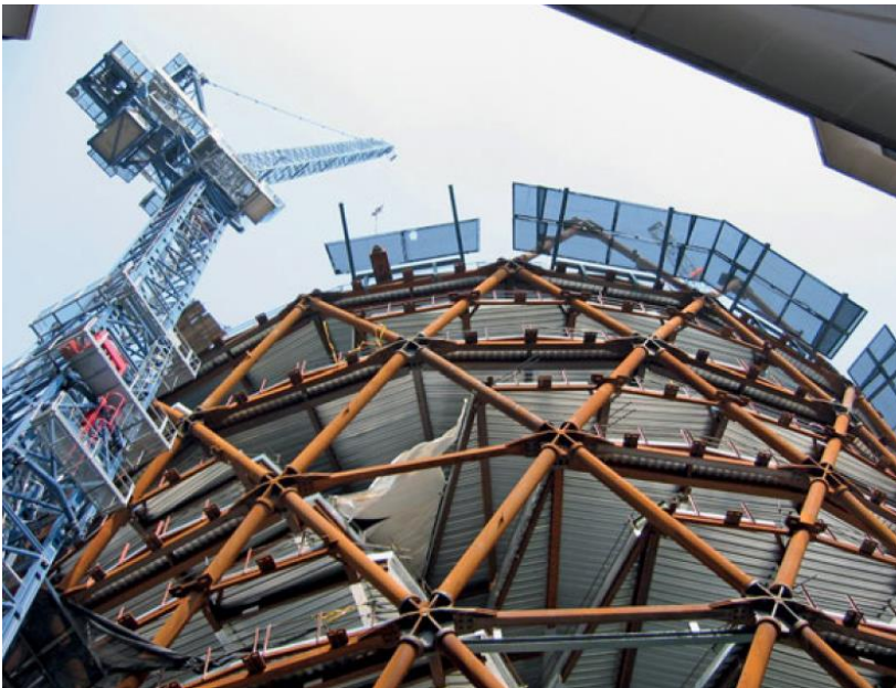
Figure 118: The horizontal rods connecting the nodes and resisting the forces arising from the curved shape
