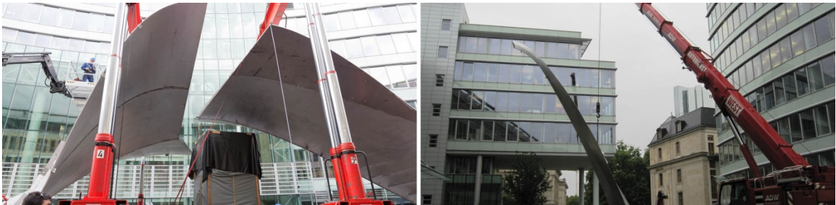
Figure 14: On site construction of the pieces with gantry cranes.
