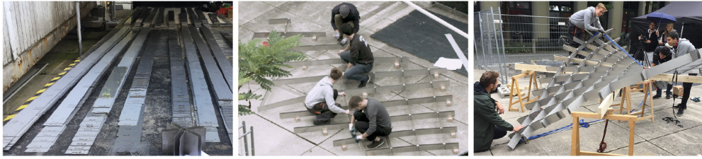
Figure 13: The straight lamellas are interlocked by hand into flat segments. The segments are then transformed elastically into their designed shape by fixing each node to 90 degrees. Nine of these segments were prefabricated off site. (Images: Eike Schling)
