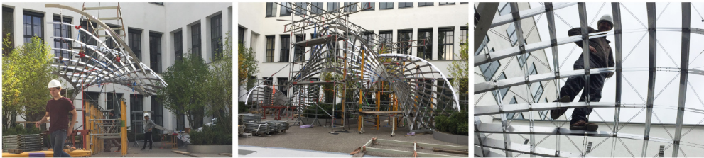
Figure 14: Installation on site. The prefabricated segments of up to 400 kg, were positioned with a crane, temporarily supported, and bolted together by hand. To activate the structural behavior of a gridshell, the completed grid is braced diagonally and fixed at supports in vertical and horizontal direction. (Images: Andrea Schmidt)
