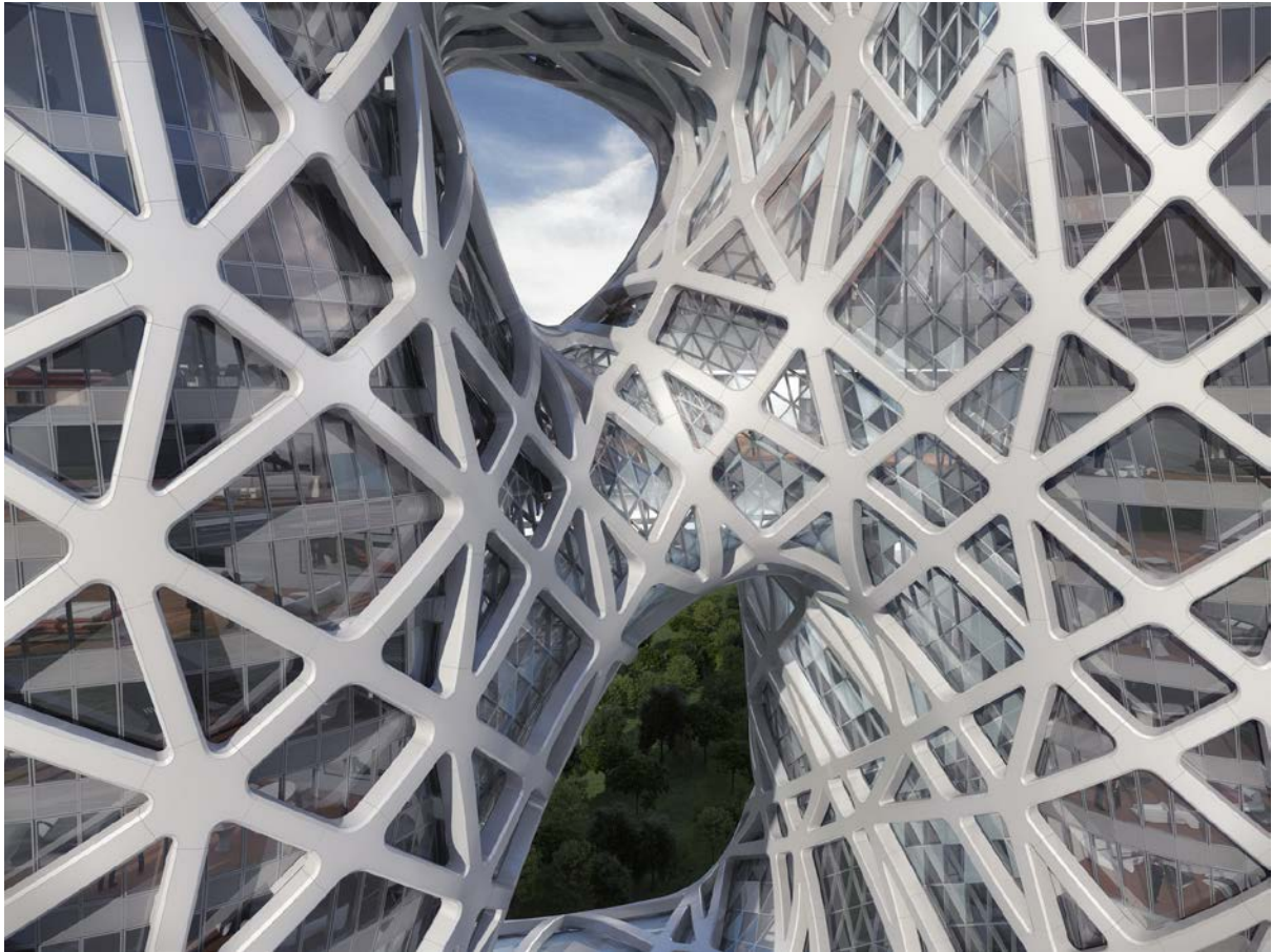
Figure 10 Free-form opening of the Morpheus Hotel. Note the curving exoskeleton and skewed and triangulated glazing. Picture Credits: Zaha Hadid Architects, Melco Crown Entertainment while the remaining facades are flat except for the single-curved edges of the block. The free-form facade's glazing is flat: Single-curved areas are approximated with skewed quadrilaterals and double-curved areas are triangulated. An exoskeleton with around 2 500 steel members supports the facade. In the free-form area, the exoskeleton's structural steel is single-curved and clad with 24 577 aluminium panels, most of which are doubly curved. Unless indicated otherwise, the information in the below sections stems from (Muscettola et al., 2017).
