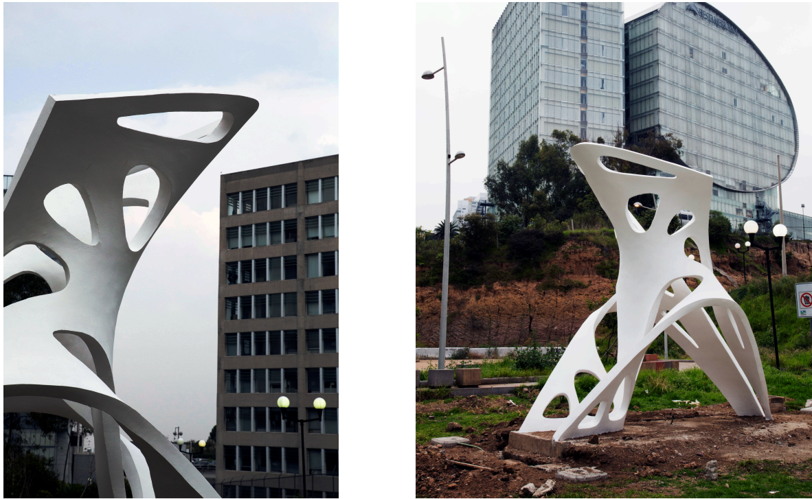
Figure 15: Topology optimized shell prototype 4 x 5 x 2m, 8 cm thick
