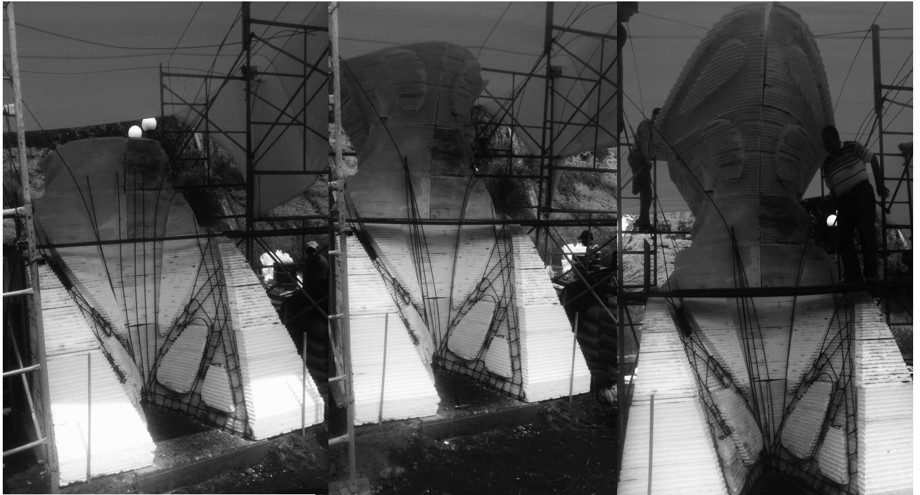
Figure 13: On site assembly of the formwork with scaffolding towers to the sides and placing of the reinforcement bars
