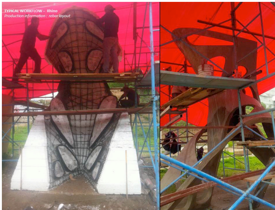
Figure 14: (left to right) Perimeter edges cover with reinforced wire plastic slip. Piece after concrete was poured and formwork removed.
