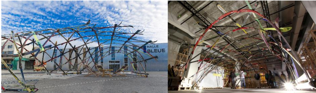
Figure 2. The ski pavilion: second assembly in the courtyard of the Blue Factory, Fribourg CH, on the left; fourth assembly in La Sucrère for the “Biennale Architecture Lyon” FR, June 2017, on the right. From left to right, three ballasts replace the connecting ropes and constrain the position of the three ground edges.
