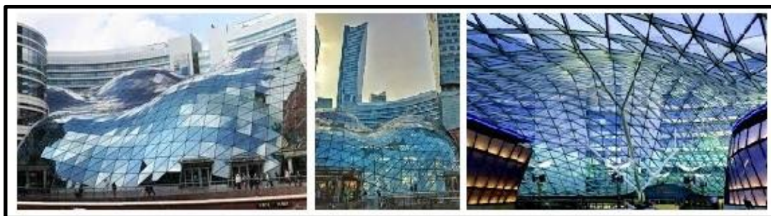
Figure 15. Blob grid-shell form of Złote Tarasy Complex Building in Warsaw [27].
