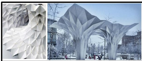
Figure 12. Rigid (segmented) folding geometries and its application on Origami Pavilion in Shinto [24].
