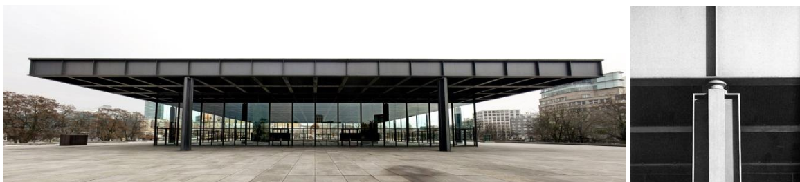
Mies van der Rohe, National Gallery, Berlin 1968. The structure is a beam grid on 8 columns with hinge joints. In both examples the modern structural principles are clearly in evidence: Distinct system type, uniformity, decomposition into discrete elements with controlled load/force transmission at the joints. Yet another aspect of modern engineering becomes evident here: These principles owe their historical rationality as much to the Fordist fabrication logic of mechanical mass reproduction of standardized industrial elements like the I-beam.
