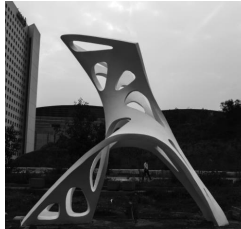
Zaha Hadid Architects' CODE group, experimental structure using a shell form as basis for the operation of the application of the topology optimization algorithm. Mexico City, 2013. Here the perforation pattern is a geometrically rationalized translation of the topology optimization.
