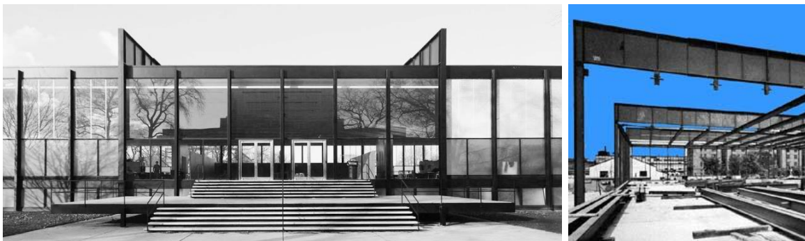
Mies van der Rohe, Crown Hall, Illinois Institute of Technology, Chicago 1956. The primary structure here uses the portal frame as distinct structural system type. A sequence of our large-span portal frames - bound together by secondary beams – make up the structure.
