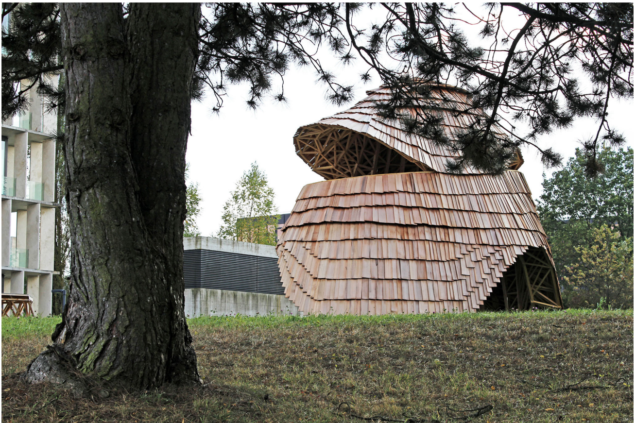
Fig. 14 Exterior image showing the shingle pattern and opening sequence of the structure
