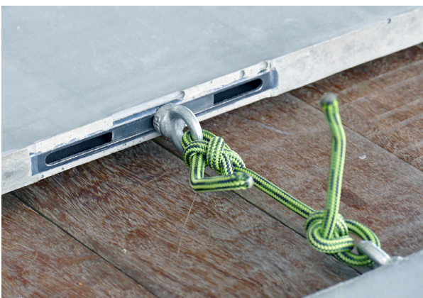
Figure 23: Thread eyes are screwed into the anchor points of the sliding device. The suspension items are ropes with running bowline hitches
