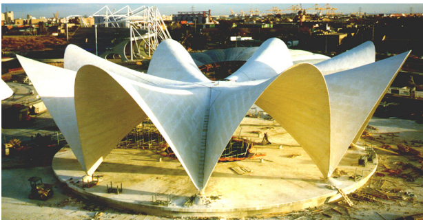
Figure 3: Oceanographic Valencia, posthumous construction after the design of F. Candela – Form passive membrane structure with compressive and tensile stresses
