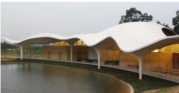
Figure 4: Crematory in Kakamigahara, Japan '06 by Toyo Ito – Freeform structure bearing compressive, tensile and bending stresses
