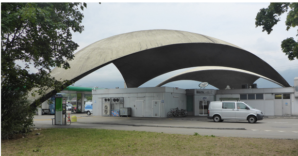
Figure 2: Service station in Deitingen '68, Switzerland by Heinz Isler – Form passive and compressive only structure
