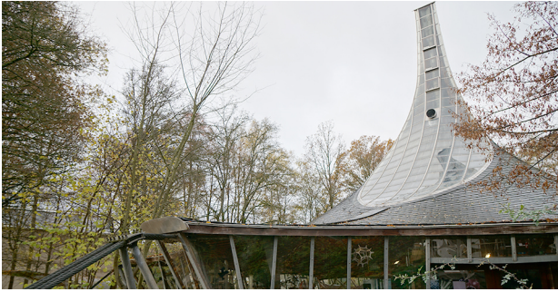
Figure 1: ILEK, Stuttgart, Germany by Frei Otto – Form active and tensile only structure
