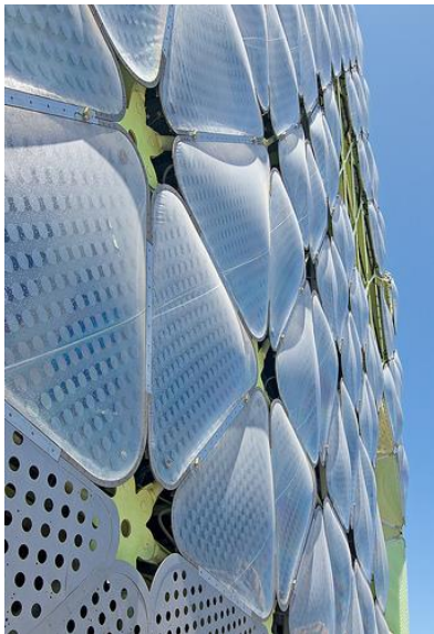
Figure 27. Smart envelope comprised of ETFE encased solar-activated lamella shades developed for the Media-TIC building in Barcelona, Cloud 9 Architects, 2011, figure adapted from dezeen.com
