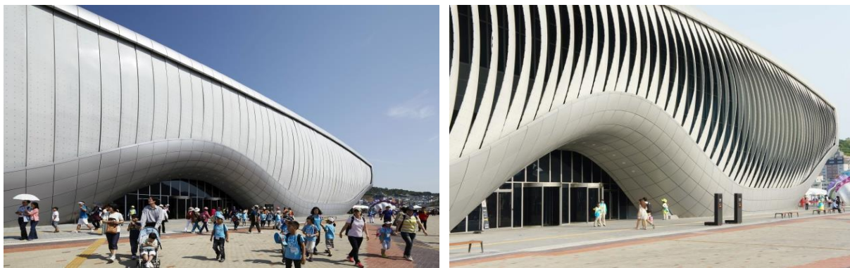
Figure 36. Kinematic façade of the Thematic Pavilion EXPO 2012 in Yeosu, South-Korea. Lef: closed Lamellas, Right: Open Lamellas, Architects: soma-architecture, Vienna; Engineer for Kinetic Façade: Knippers Helbig, Stuttgart, New York, Photo adapted from e-architect.co.uk.
