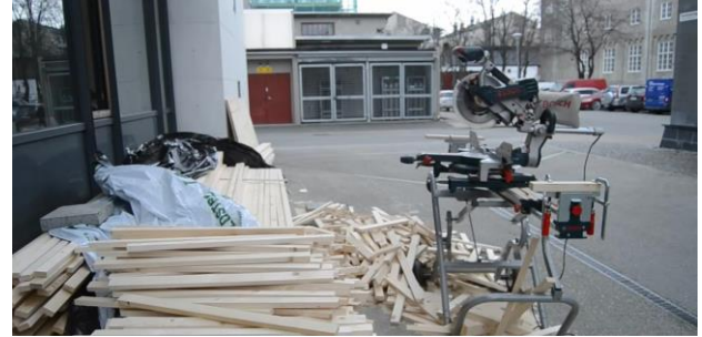
Figure 13: Cutting the segment. The pile on the right shows the lengths of the waste.
