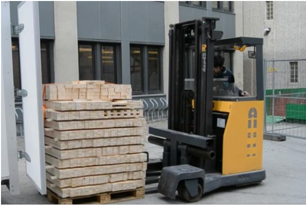
Figure 15: ½ of the complete gridshell stacked on one pallet
