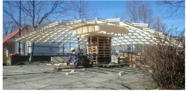
Figure 19: From the erection process. The pallet tower in the centre is incrementally heightened. The border was always approximately 1200 mm from ground level
