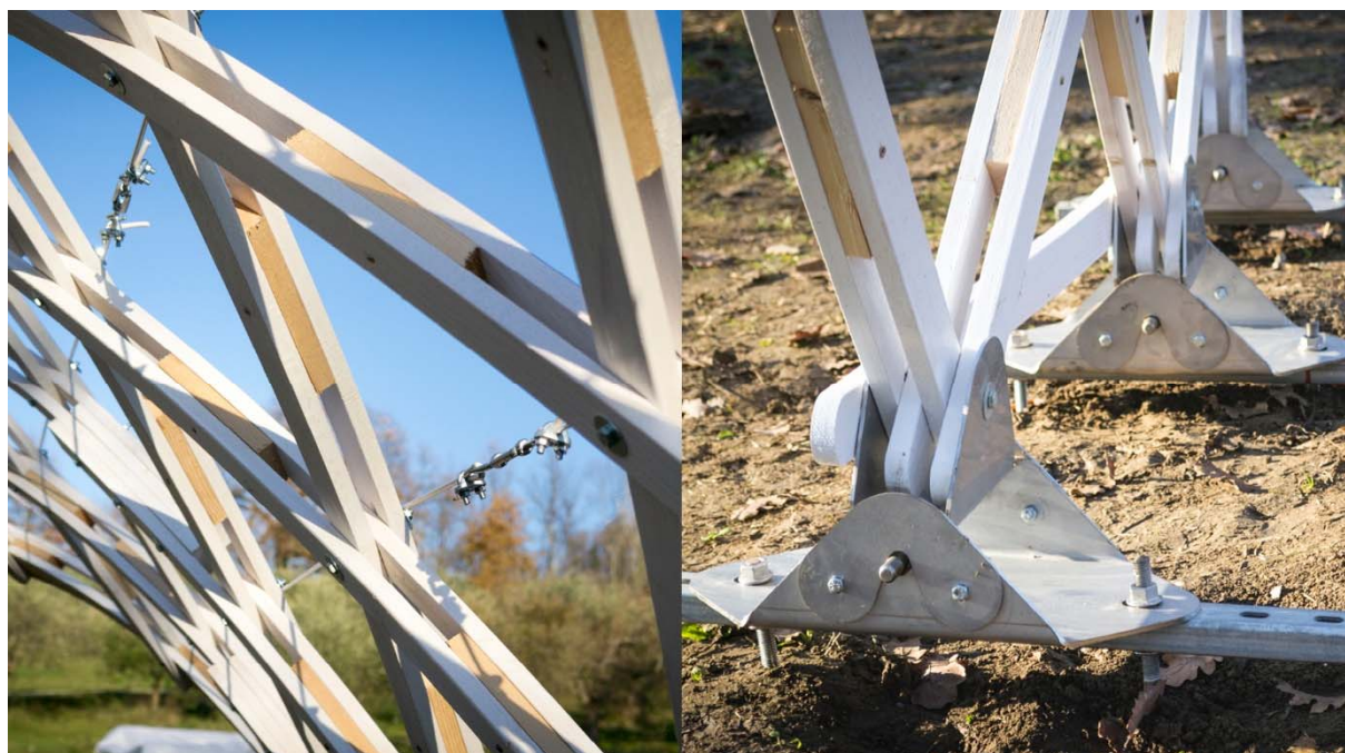
Figure 7: details of the diagonal bracing and shear blocks (left), ground connection (right). [Image: A. Liuti]
