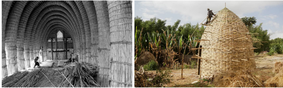
Figure 2.2: Vernacular bending-active structures – ( left ) Traditional mudhif collective house by Madans people in Iraq, ( right ) traditional hut by Dorze people in Ethiopia.
