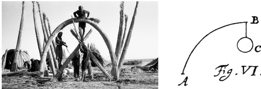
Figure 1.4: Bending as a self-forming process – (right) Construction of a traditional mudhif house from plant stems (Iraq) and (left) Elastica curve by Euler (Euler 1744)
