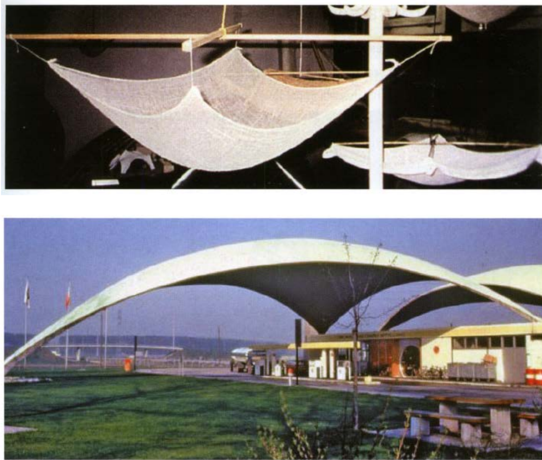
Figure 20: Forces and Forms are correlated - Heinz Isler, Service Station in Deitingen (Arturo Tedeschi, 2014).
