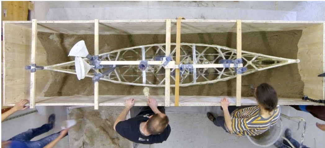
Figure 5.15: The canoe formwork was placed in a simple box that was simultaneously being filled with sand while concrete was being cast inside the formwork (dbt, PCBM, ETH Zürich, 2017)
