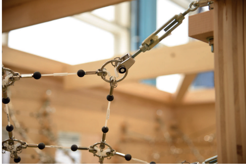
Figure 13.2: Turnbuckle connecting the cable net structure to the boundary node at the wooden frame and realization of a node in the net as ring construction with attached rods and with markers for the image-based measurements.
