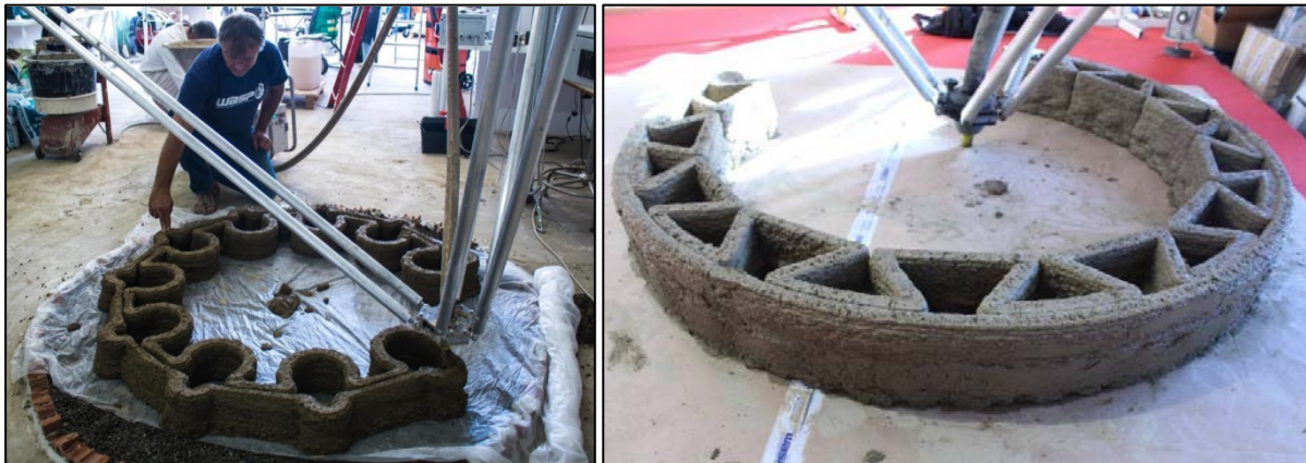
Fig A.30 – WASP 3D printing clay structures (Krassenstein, 2014)
