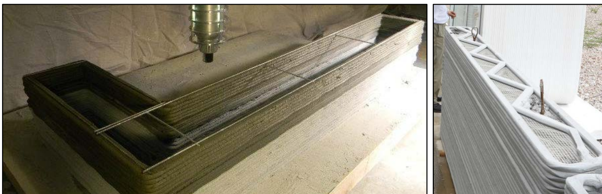
Figure 1.2 – 3D printed walls by TotalKustom (left) and Yingchuang (right) ( totalkustom.com , 2014), (Yingchuang, 2015)
