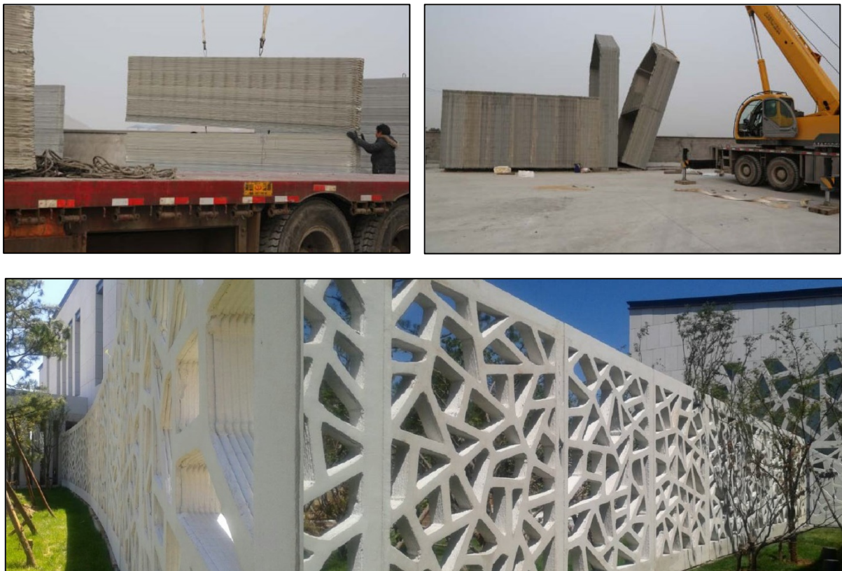
Figure A.22 – Top: Transport and assembly of printed components, Bottom: printed wall element (Yingchuang, 2015)
