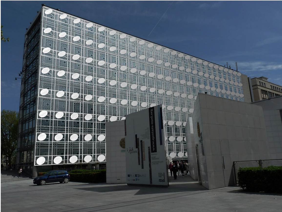
Figure 64- Schematic illustration of sun-tracking modules on Jean Nouvel's Arab world institute building in Paris. Image source: http://www.greatbuildings.com/cqi-bin/qbi.cqi/L_Institut_du_Monde_Arabe.html/cid_3027883.jpg , illustration by the author
