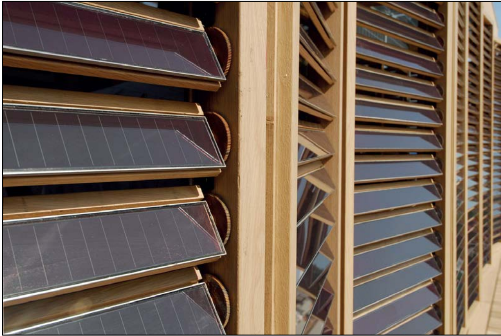
Figure 5- Intelligent façade of automated wood louvers with building integrated photovoltaics create a continuous façade for TU Darmstadt's 2007 Solar Decathlon House
