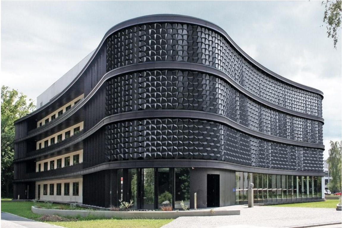
Figure 1-4: Flare Façade – The modular façade is composed of metal flake elements that are controlled by a series of pneumatic cylinders. These elements reflect sunlight in a way that casts a shadow on some of the faces of each element, giving them darker colors. The façade does not optimize the energy performance of the indoor spaces, but socially interacts with people outside the building and operates as an interactive piece of art. 15
