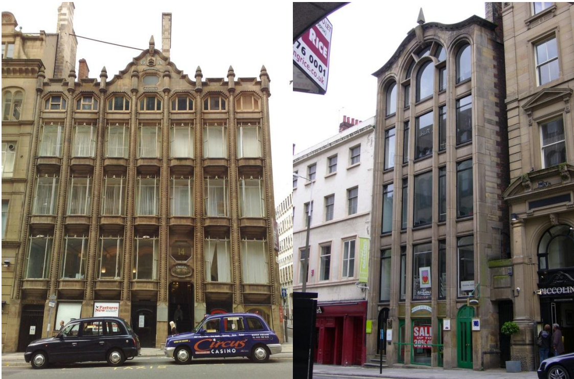
Figure 1-1: Curtain Walls – The left image shows one of the world’s first curtain walls in England, Oriel Chambers. The right image shows a building by the same architect, which also has a curtain wall system, built two years later. At this time, the amount of glazing used was large compared to adjacent buildings in the area. The architect’s goal was to allow more daylight penetration into the space, as a means of energy-saving. 1
