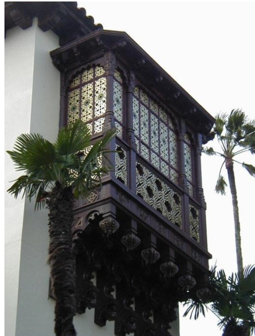
Figure 2-4: Egyptian Mashrabiyya – the Mashrabiyya is a great example of an environmental façade treatment for optimizing daylighting, minimizing glare, and driving cool air into the space. The image on the left 34 shows the indoor effect of this element, while the image on the right 35 shows the exterior look of this ornamental Egyptian icon.
