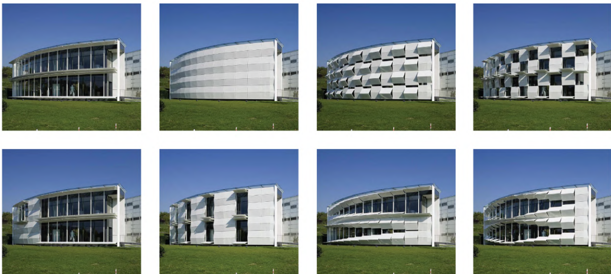
Figure 3.3: Different façade configurations for the Kiefer Technic Showroom. Ernst Giselsbrecht + Partner, Graz, 2007 (source: https://www.e-architect.co.uk/austria/kiefer-technic-showroom ).
