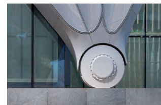
Figure 3.9: Close-up of The Shed's bogie wheels (source: https://artsummary.com/2019/04/05/ ).
