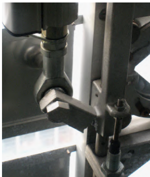
Figure 6.16: Mechanical diaphragms of the Arab World Institute – damage to the arm that transmits the force of the motor to the diaphragm actuation mechanism (source: Meagher (2015)).
