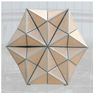
Figure 3.17: Shading panels for the Al Bahr Towers (source: https://www.arch2o.com/al-bahr-towers-aedas/ ).
