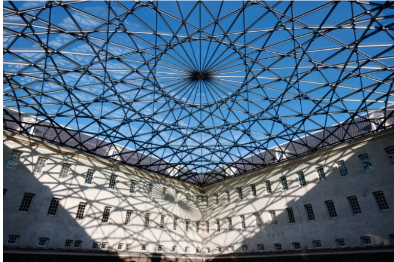
Figure 2.7: View of the grid shell at the Dutch Maritime Museum. Figure taken from [14]
