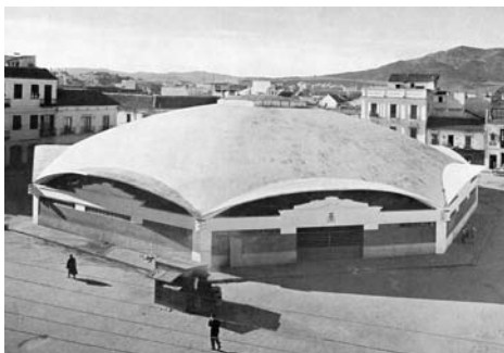
Figure 2.7 Market hall in Algeciras, Spain by Eduardo Torroja from 1933 spanning of 47,6 m, to the time largest spanning spherical shell
