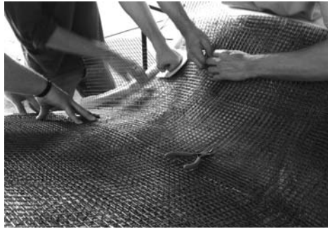
(b) ...and tailoring to fit into the formwork without damaging foam surface
