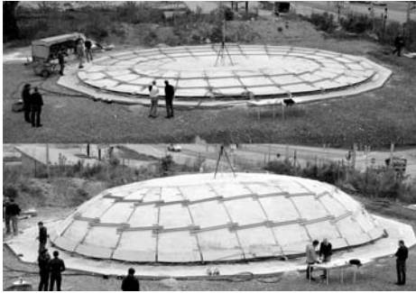
Figure 4.13 Pneumatic forming of hardened concrete ©TU Vienna
