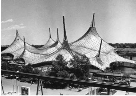
(a) Form active and solely tensile structure—German Pavilion Expo 1967, Montreal, Canada by Frei Otto, ©ILEK, University of Stuttgart
