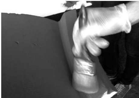
(c) Concrete contact areas are coated with a special lacquer and release agent
