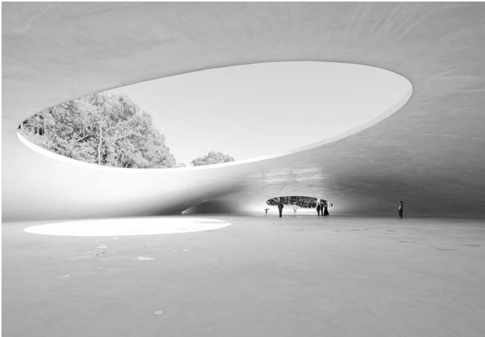
(c) Teshima Art Museum, Japan by Ryue Nishizawa and Rai Naito ; concrete shell cast on earthen formwork. Photo: Iwan Baan
