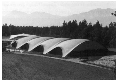
(d) Tennis courts , Heimberg, Switzerland, 1979. The four adjacent shells are derived from inverted hanging models, with a shape following the flying-line of tennis balls
