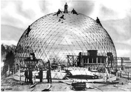
Figure 2.4 Planetarium in Jena by Dischinger and Bauersfeld from 1922 with a diameter of 16 m. The assembled steel grind facilitates the accuracy of the spherical geometry
