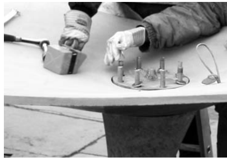
(c) ...and fixed with screw end nuts from the top of water drain
