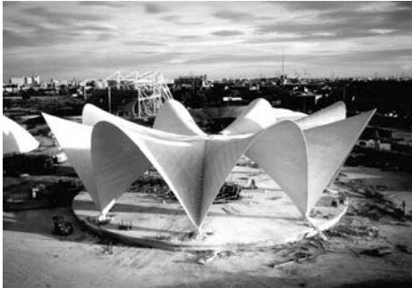
(c) Form passive membrane structure with compressive and tensile stresses—Oceanarium Valencia, posthumous construction after the design of Félix Candela, ©CMD Ingenieros
