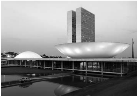
(a) National Congress, Brasilia by Oscar Niemeyer ; built with formwork made of wooden planks.
