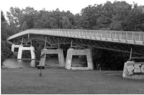
Figure 4.4 The Gärtnerplatzbrücke in Kassel is a pilot project with glued UHPC construction elements
