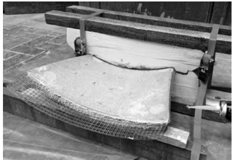
(d) Closed formwork for the casting of the joint
