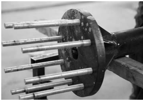
(c) Embedded steel pipe with screwed connection at the column head
