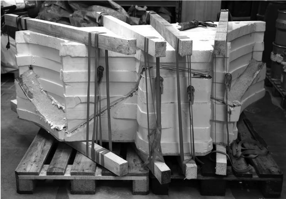
Figure 5.19 Closed formwork for one concrete element of Möbiusban(k)d ready for concreting
