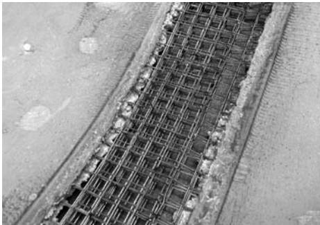
(c) Overlapping reinforcement in the joint; implemented ridges at the border of the segments
