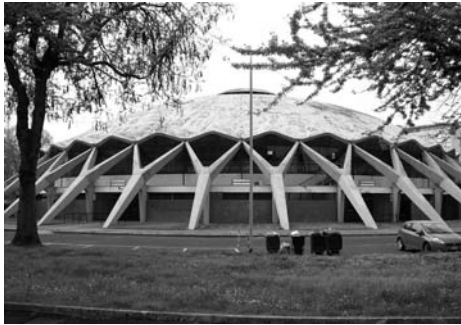
(a) Shell stresses are transferred by inclined Y-shape buttresses to a prestressed concrete ring below ground to bear the horizontal shear
