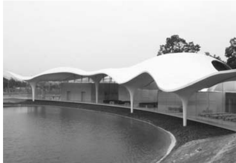
(d) Freeform structure with compressive, tensile and bending stresses—Crematory in Kakamigahara, Japan 2006 by Toyo Ito, Photo: Toyo Ito & Associates, Architects
