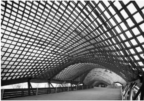
Figure 4.18 Multihalle in Mannheim 1975 by Frei Otto . A network of wooden strips has been pushed into shape and locked at the intersections
