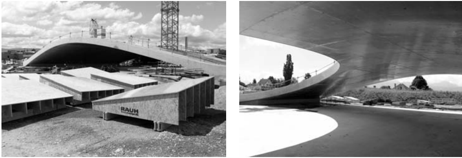
Figure 4.9 Wooden formwork elements used for the double curved concrete shell of the EPFL Rolex Learning Center in Lausanne by SANAA , ©B+G
