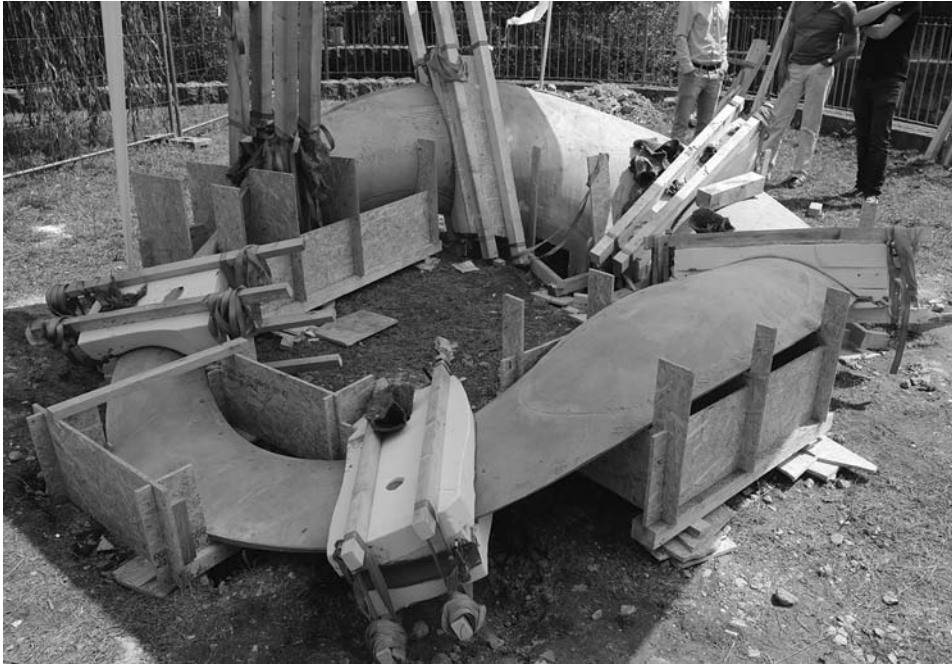
Figure 5.22 All connection joints of the shell structure in their formwork, just after concreting
