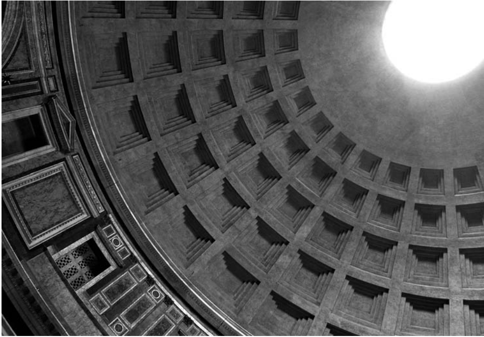
Figure 4.1 Inside view of the rotunda in the Pantheon in Rome. The spherical cupola is built with Opus Caementitium
