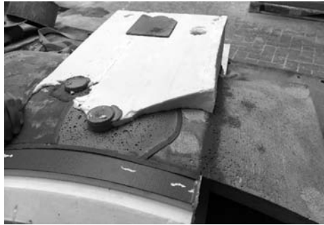
(b) The concrete of the joint casting leaks slightly out of the formwork
