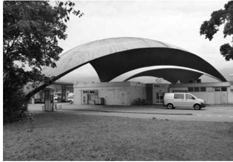
(b) Form passive and solely compressive structure—Service station in Deitingen 1968, Switzerland by Heinz Isler
