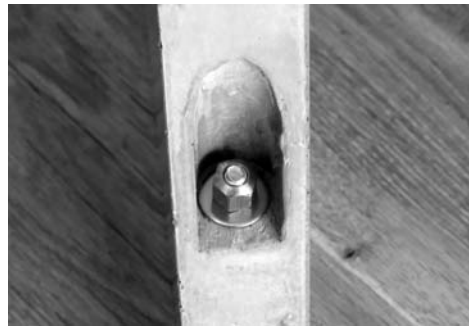
(c) Threaded bar end and mounting nut
