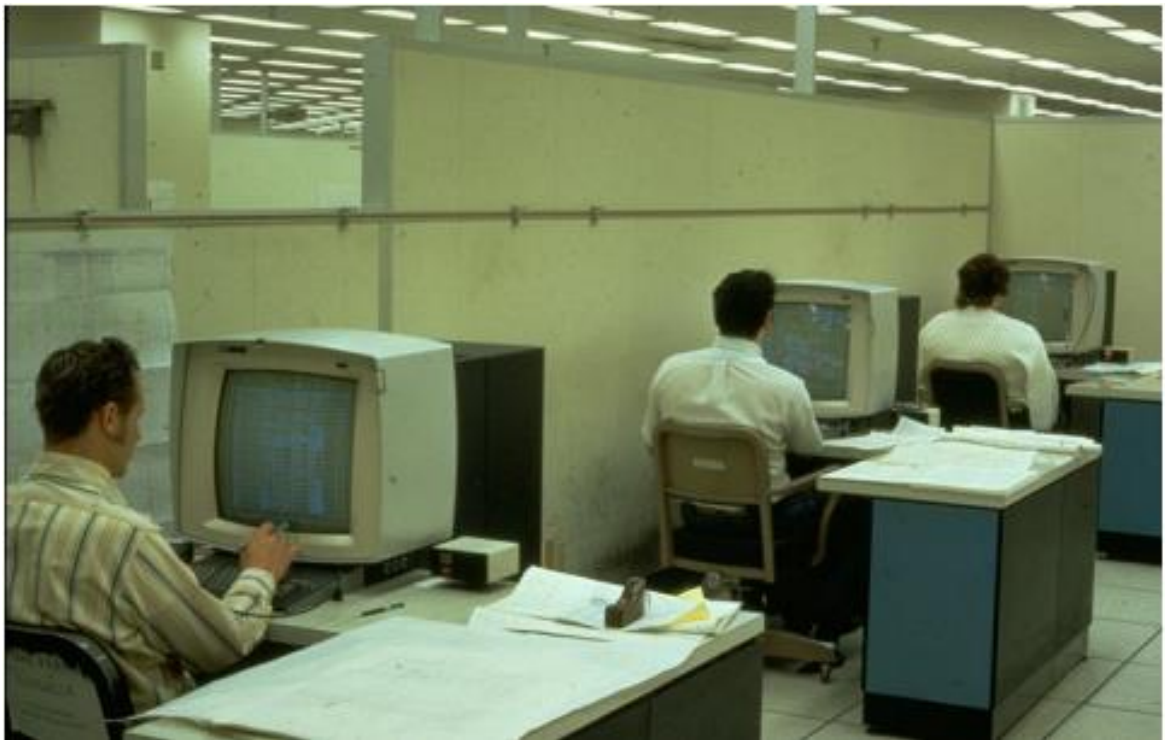
Figure 2-5 The IBM 360 Computers with the 2500 graphics display terminals, located at Lockheed Engineering Department (Weisbery, 2008).
