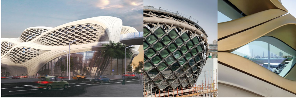
Figure 2: Geometrical complexity in a glazed building envelope, King Abdullah Financial District Metro Station in Riyadh, designed by Zaha Hadid Architects. Exterior rendering (left), construction of façade diagrid (middle, photograph by Faisal Bin Zarah) and close-up of detailed facade mockup (right) (all images property of RDA and courtesy of ZHA).
