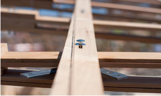
Figure 2.13: Pavilion ZA: typical connection showing thinner laths used for higher curvature areas at entrances, slotted hole and steel bracket for bracing attachment (image – AStA Cluj)
