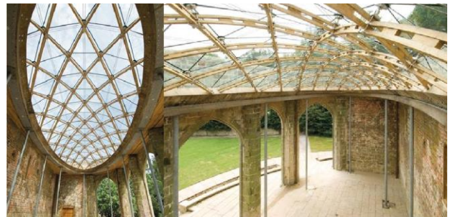
Figure 2.8: Chiddingstone gridshell; interior view; detail of grid layout showing two layers, nodal connector and shear blocks (from [7])
