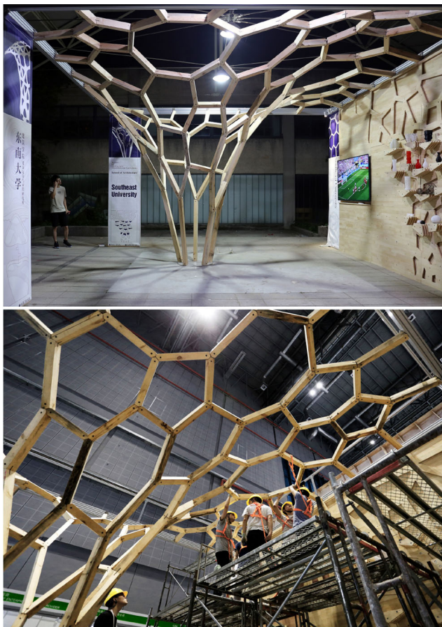
Fig. 13 The Upsilon pavilion as a timber Voronoi shell
