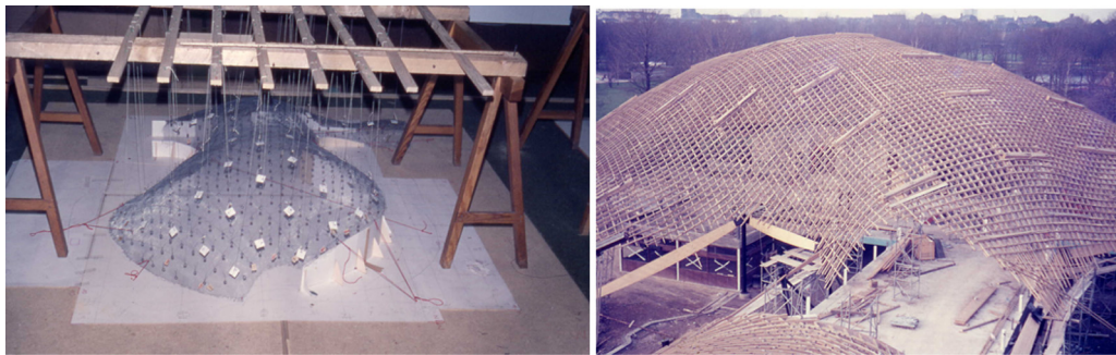
Figs. 10 & 11. Model of lifting positions and arrangement on site.
