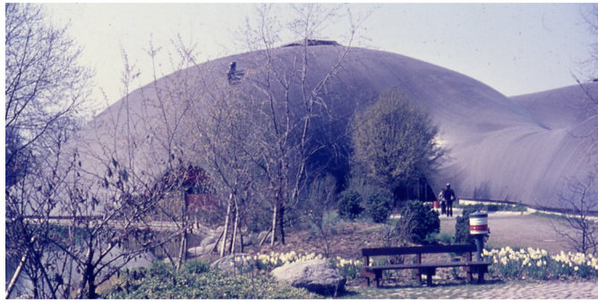
Fig. 12. The gridshell covered with dark but translucent PVC coated mesh fabric.
