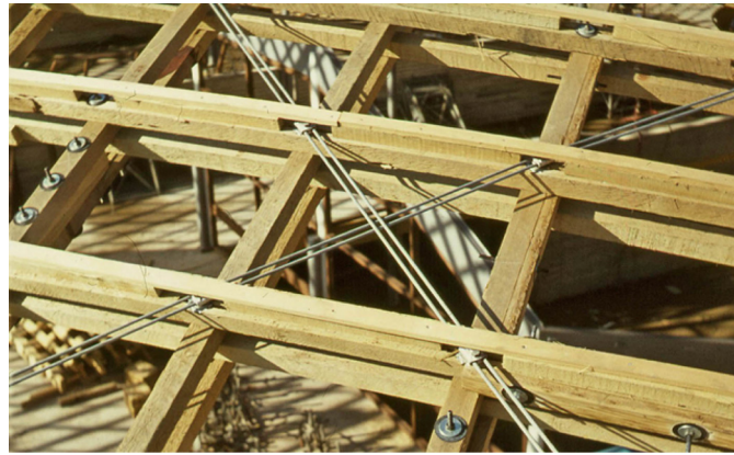
Fig. 6. Detail of grid construction.
