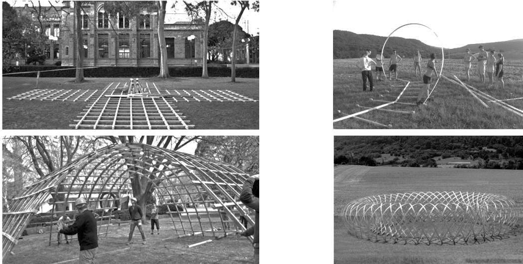
Figure 1.1 – Left: Site-sprung gridshell. Source: www.karamba3d.com . Right: sequentially erected elastic timber gridshell. Source: coda-office.com .
