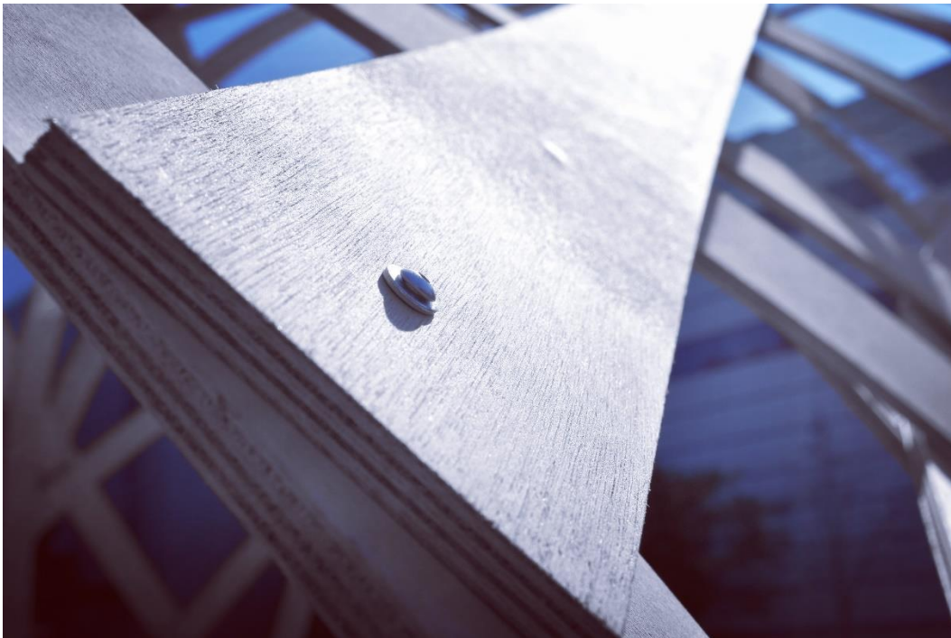
Figure 5.10 - Rotational joint connecting 2 laths. Photo credit: Heidi Erickson.
