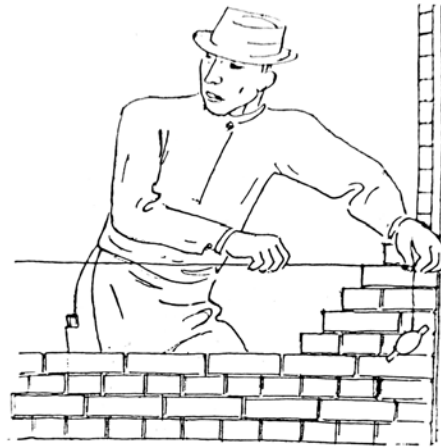
Figure A.5: The bricks should all be level in the horizontal direction. The most common way to achieve this is to use string that is attached between to rods.[31]
