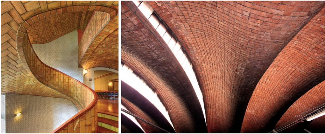
Figure 1.2: To the left a staircase by the Guastavino company showing both structural and geometrical complexity achievable using brick vaults[7]. To the right the roof construction on Cítricos Caputto fruit packing plant , by Dieste [48].
