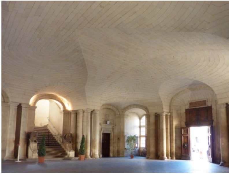
Figure A.19: The stone vault at Hotel de Ville by Jules Hardouin Mansart is a famous example of stereotomy in architecture [49]
