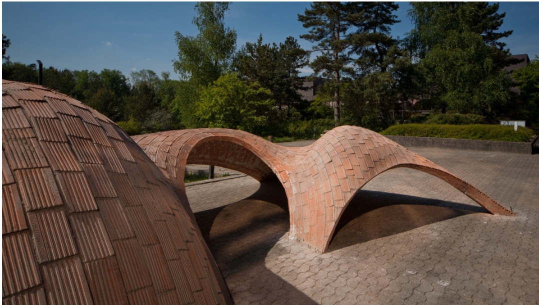
Figure 1.3: A free-form compression shell that was developed and built by the Block Research Group at ETH in Zurich [43].
