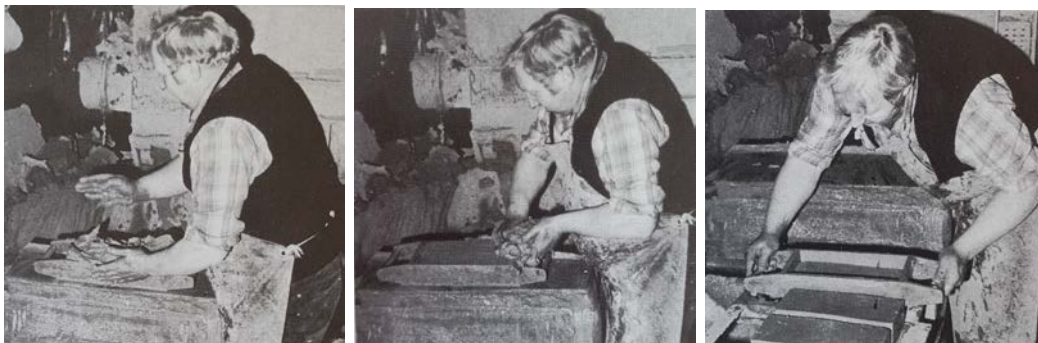
Figure A.1: A traditional method of brick making is by putting it into wooden forms. Today this is not very common and the bricks are usually pressed by a machine. This method gives the brick marks of the form and also results in some deformation and transformations from the cuboid. The deformations is in general not a problem due to the adaptability for tolerances of the mortar joints. This method is more in line with traditional brick making then the wire-cutting method. [30]
