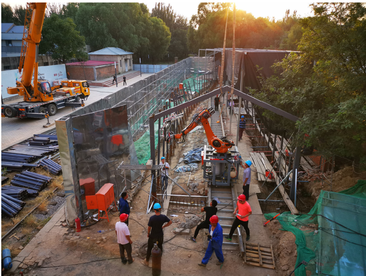
Figure 14 Industrial Robots for On-site assembly of Steel Structure
