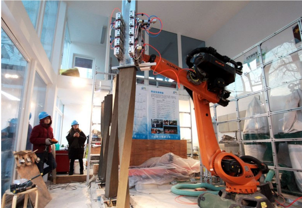
Figure 5 Dynamic concrete casting and slip-forming process
