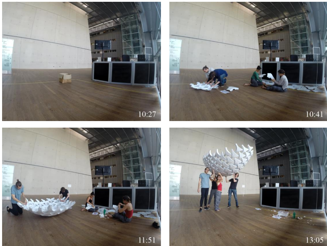
Figure 11: Demonstration of the rapid assembly of the pavilion.
