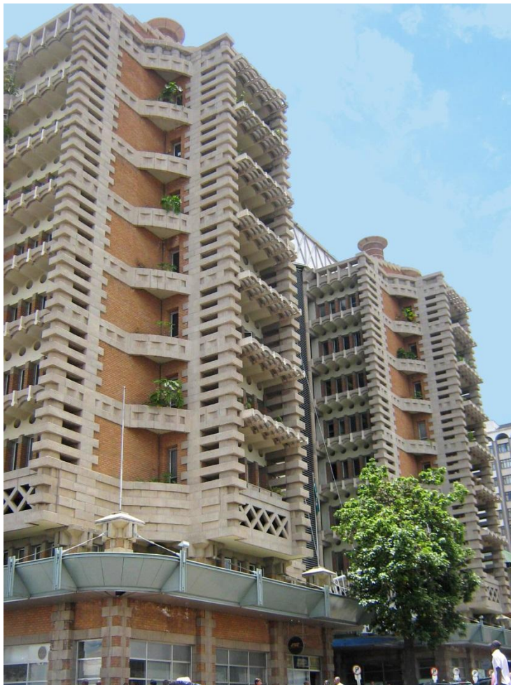
Fig. 94 The Eastgate Center- a building inspired by termite mounds that maintain comfortable conditions close to the equator without mechanical cooling. ( Ibid )
