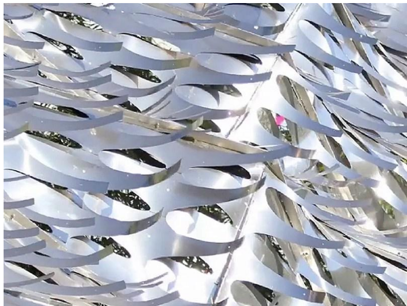
Fig. 95 Sun shade canopy made from thermo bimetal. (CO.DESIGN, 2012, http://www.fastcodesign.com/1671279/a-shape-shifting-heat-sensitive-metal-lets-buildings-breathe )
